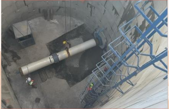
600mm (24") Pipeline in Concrete Sleeve Beneath A1
