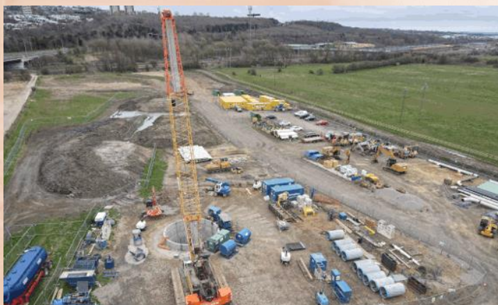
Aerial View of Site Works
