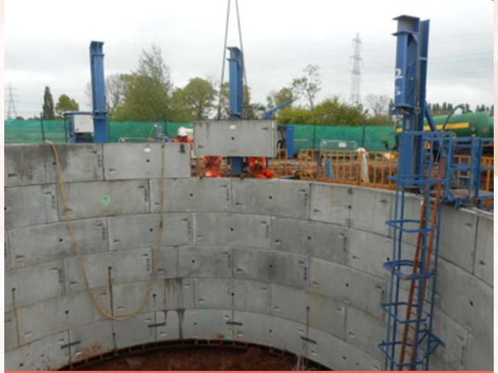
Construction of Caisson Shafts Using Hydraulic Jacks
