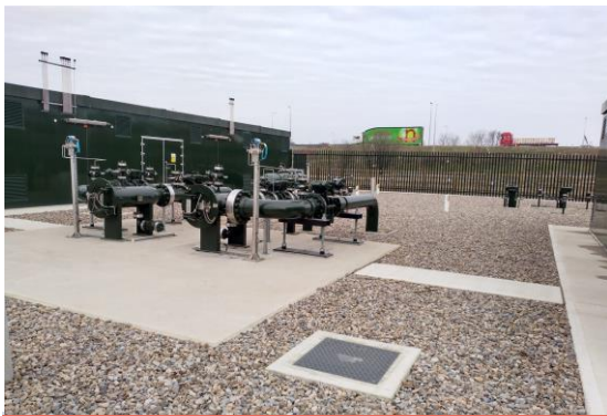
AGI Compound & Pipework
